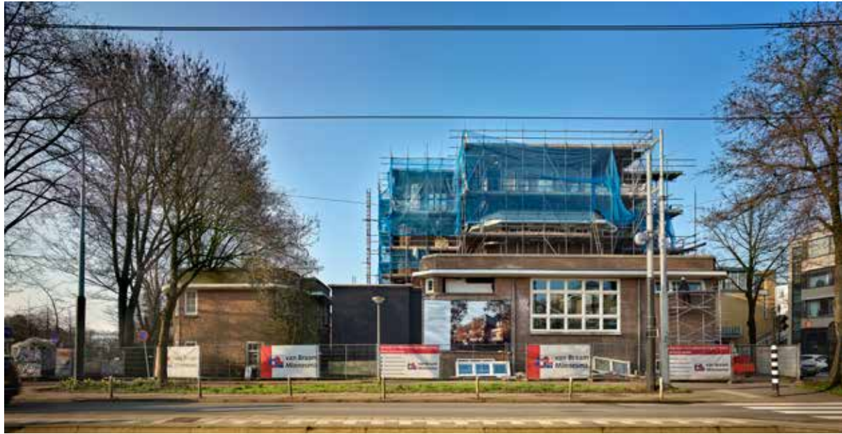
A rooftop structure was added, increasing the building's height by about one and a half times
